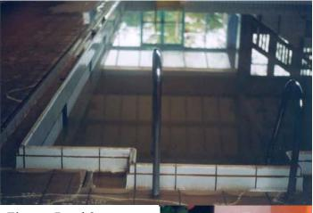
Figures 7 and 8: The swimming pool in Tonbridge, built in a flood-vulnerable area against the EA's advice and flooded. The layer of mud left inside (above) led to indefinite closure (right).
